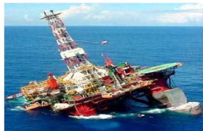
d) Platform P-36 accident, 2001
