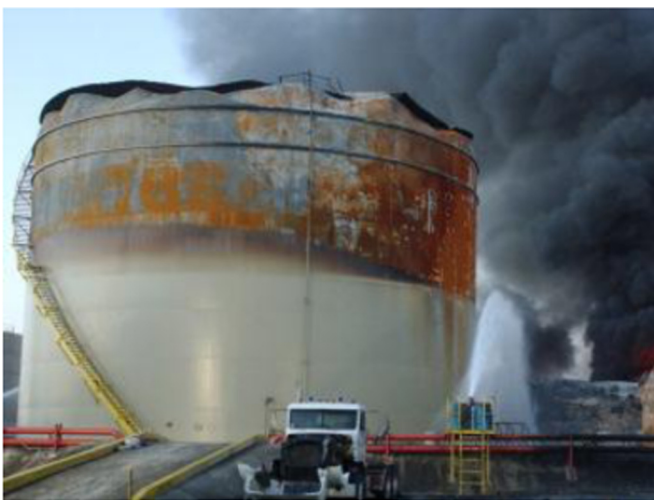
Fig. 3. Tank that was affected by a fire [1].
