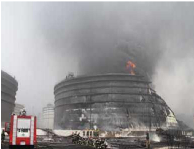
Fig. 2. Accident scene of tank explosion.
