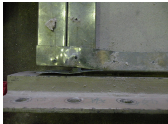
Fig. 5. Tearing failure of bottom track (FC-C09-HT-2).
