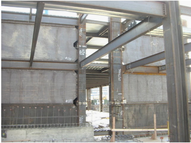
Fig. 1. SPSWs in practical construction.
