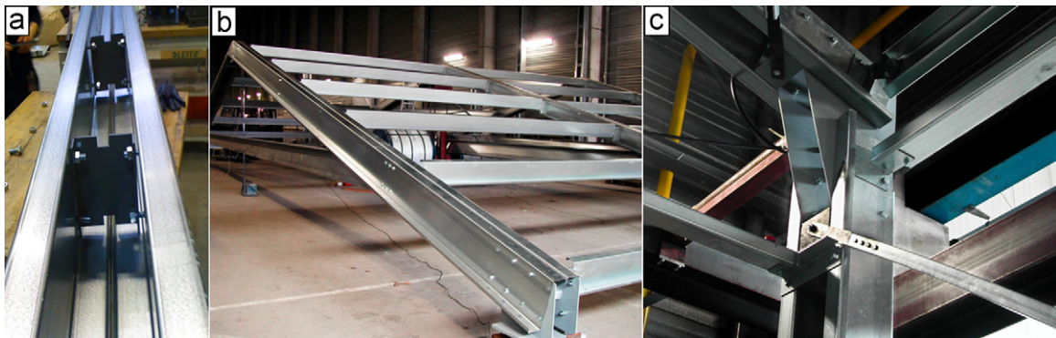
Fig. 2. Double-Z built-up CFS members: (a) assembly and intermediate spacers; (b) and (c) roof and eave joint in structures from Z-profiles.
