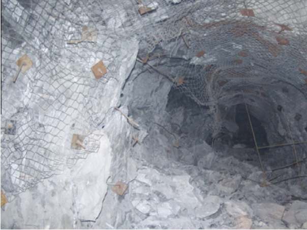
Fig. 1. Stress-driven failure near the boundary of an excavation.
