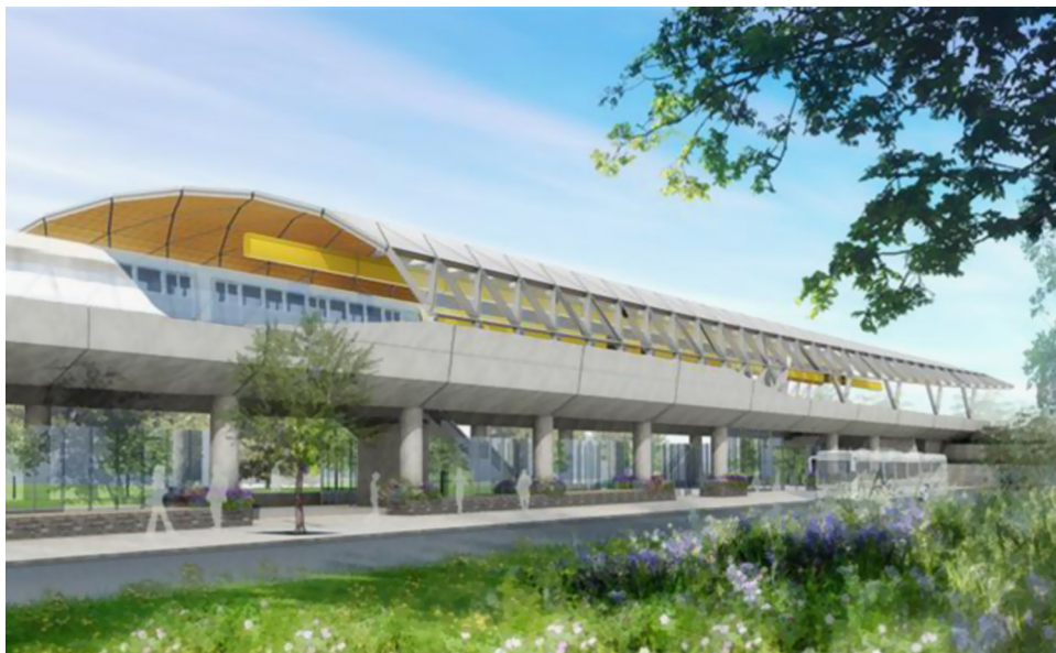
Fig. 2. Station 1 along the Rideau River in Ottawa, Canada (Ottawa Light Rail Transit (OLRT) ( http://www.ottawalightrail.ca/en/ )).
