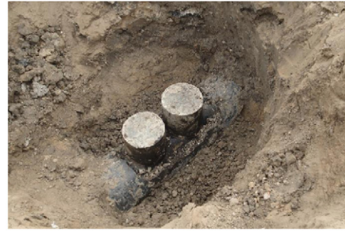
Fig. 3. Drilled holes had been repaired by welding hats.
