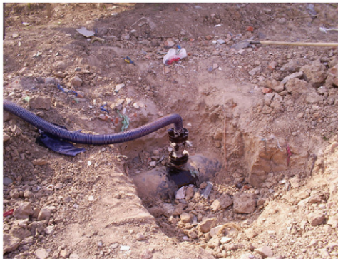
Fig. 2. Illegal valves and hoses installed in the pipeline by stealers.
