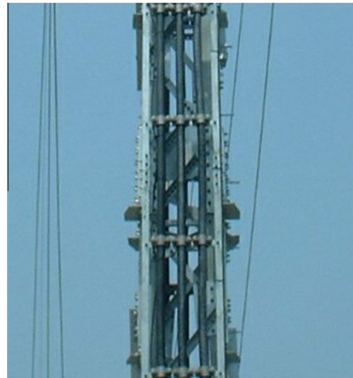
Fig. 3. Lateral view of a junction tower.
