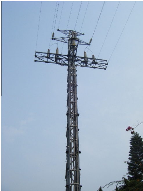
Fig. 2. Junction tower with structural steels.
