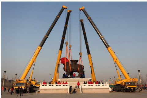
Fig. 1. Multiple mobile cranes.
