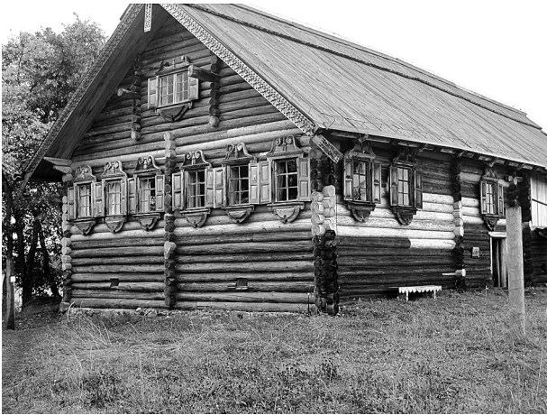
Fig. 1. Numerous new patches influenced the aesthetic appearance of the house of peasant Sergeev from the Village of Logmoruchei (1910), Kizhi Open-air Museum, Russia.
