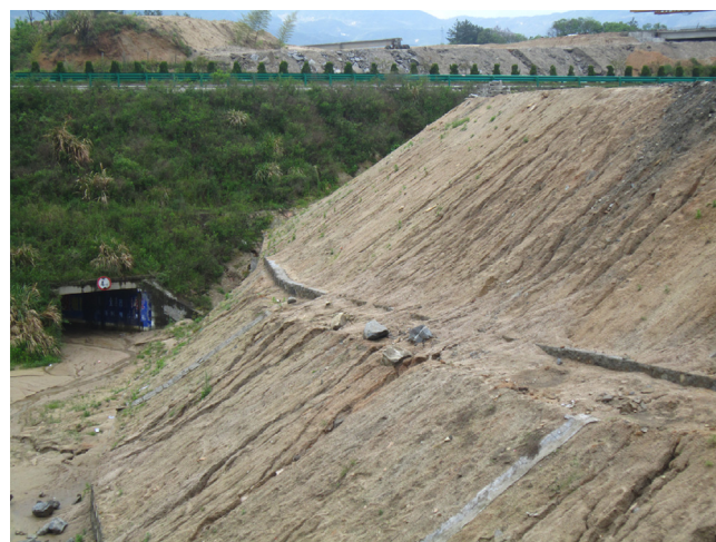
Fig. 1. Distance view of the unrestored highway slope.
