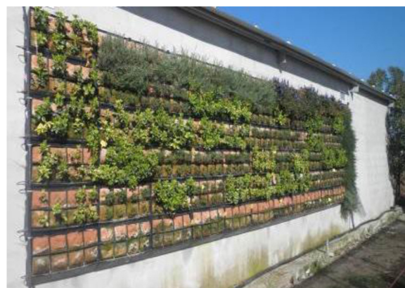
Fig. 1. Vertical garden in the wall overlooking the water feed pipe on the left side of the plant cell wall.
