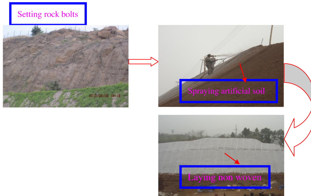
Fig. 1. The steps of hydroseeding technology.
