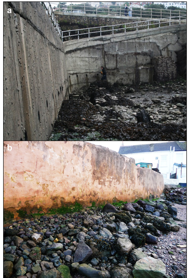
Fig. 1. Concrete coastal structures with typically vertical, relatively smooth surfaces often have limited ecological value.
