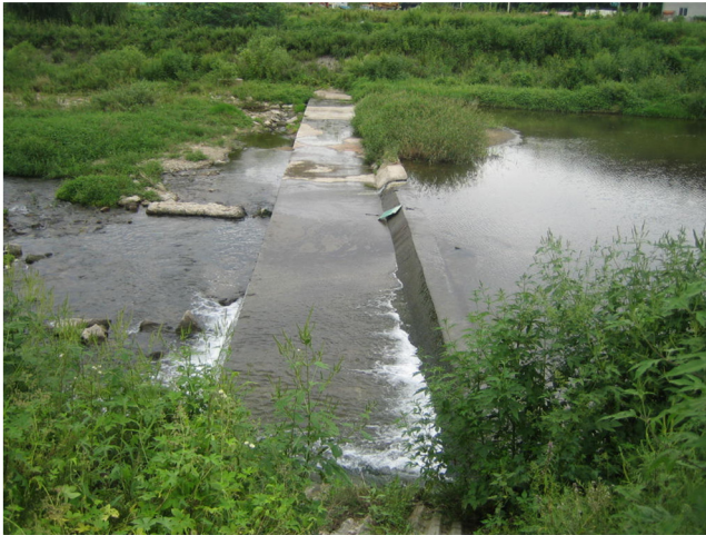
(a) Low-head concreted fixed weir
