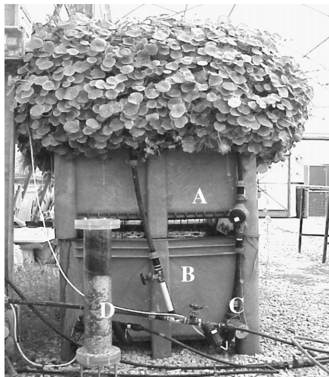
Fig. 1. Recycled vertical flow constructed wetland (RVFCW). (A) vertical flow constructed wetland, (B) reservoir, (C) recycling pump, and (D) demonstration of filter media layers (peat, tuff or high surface area plastic media, and lime pebbles in top middle and bottom layers, respectively).
