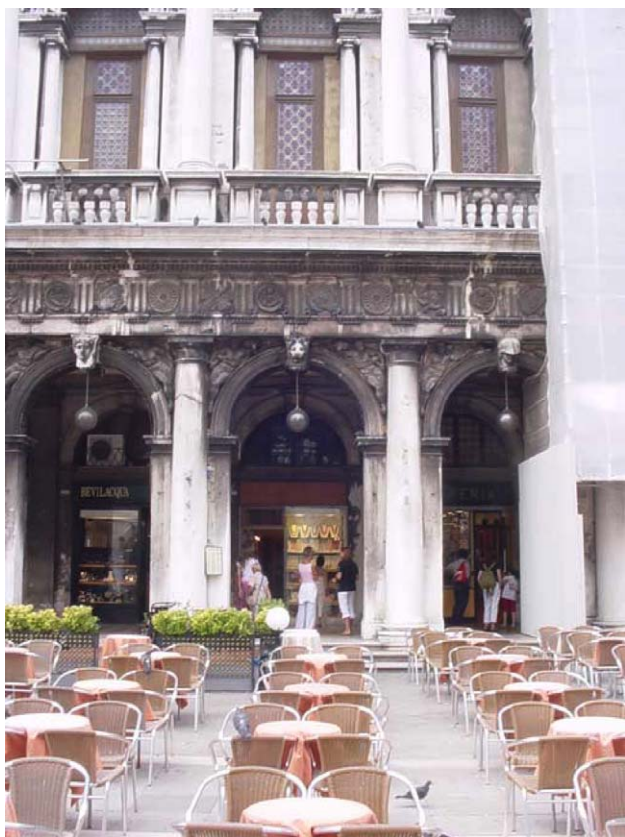
Fig. 1. The impact of BC deposition on buildings in Venice. The upper levels are more exposed to wind and rain such that the BC has been much reduced. At low levels the BC persists. Photographs taken by E. Highwood, August 2004.
