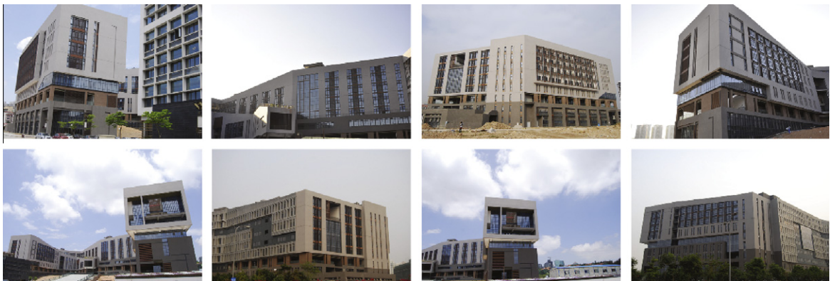
Fig. 1. An unorganized photo collection of a building, like the one shown, is sorted to quickly find camera viewpoints, create a piecewise planar model (see Fig. 2), and to facilitate fast multi-view reconstruction.
