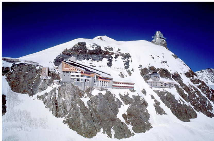
Fig. 2 – View of the buildings at Jungfrauoch. In front is the complex of the Jungfrau Railways including several restaurants and tourism facilities. To the right, the research station, which was built in close agreement to the original planning. On top the Sphinx, which is accessible by fast elevators. (Source: Jungfraubahnen).
