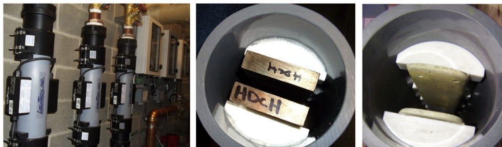
Fig. 1. Three Copper-Silver Ionization (CSI) cells with three corresponding controllers (left) treated incoming water intended for both hot and cold uses. Inside a CSI cell with "fresh" (unused) 70% Cu–30% Ag electrodes (middle). Inside a CSI cell with used electrodes (right).
