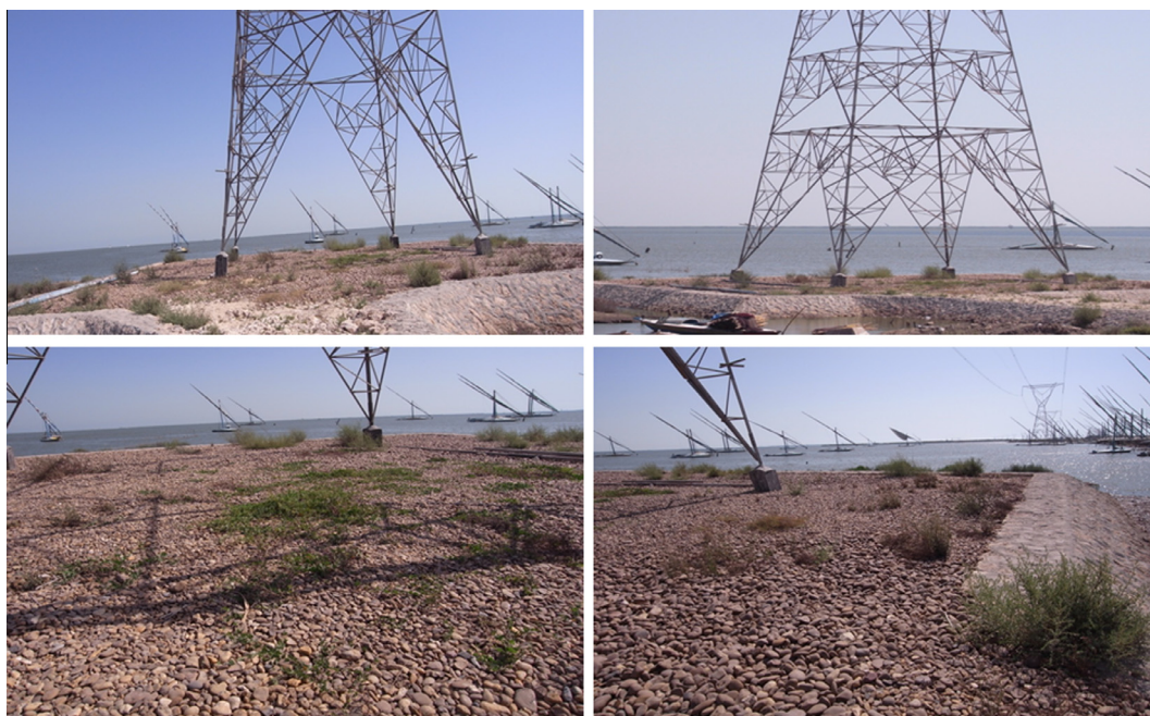
Figure 1 Photos of constructed and benched gravel pads for stabilizing powerline towers dominated by terrestrial alien plant species in Lake Burullus.
