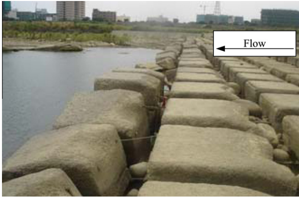
Fig. 1. Edge failure at Lung-En Weir in Taiwan (2009).
