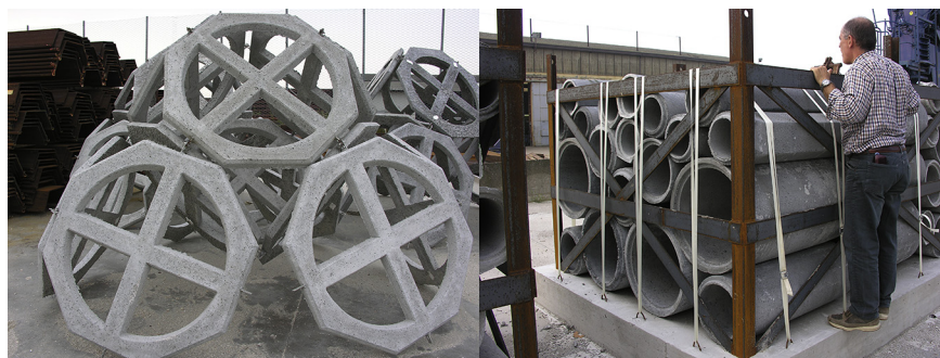
Fig. 1. Example of ARs structures deployed: pyramids of slabs (2 floors, 1.8 m height), assembled with slabs of ‘sea-friendly’ concrete (Tecnoreef®), on the left and bundles of tubes, made by common concrete, laid on a concrete slab and retained by an iron cage (1.8 m height, on the right).
