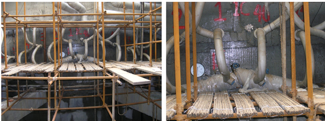
Fig. 1. The photos of freeze process and freeze pipes.
