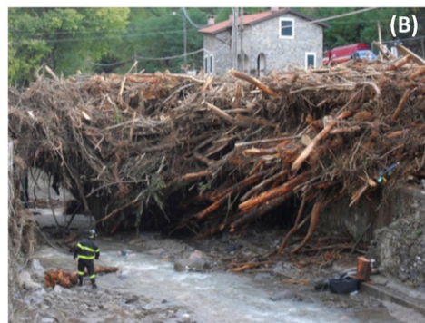
Fig. 1. The different types (at different scales) of geomorphic effects of wood in rivers (A, from Montgomery et al., 2003) have long been investigated by the geomorphological community; whereas the additional flood hazard induced by wood jams (B, a huge wood jam created by a bridge during a flood event in Italy, photo courtesy of the Province of La Spezia) has been dominant among hydraulic engineers in Europe and Japan.
