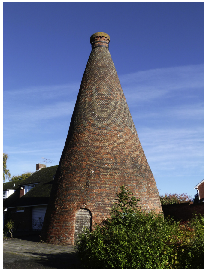
Fig. 3. The iconic up-draught bottle brick kiln at Nettlebed built in 18th century. Later in 1927 it was converted for lime burning but finally closed in 1938. It was restored to its original form in 1974.
