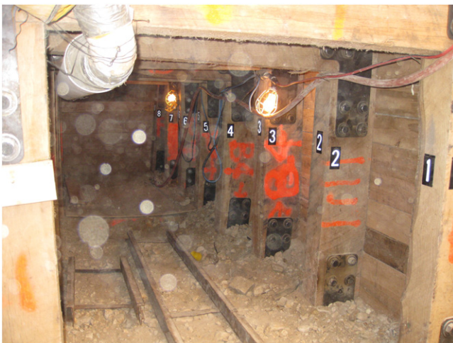
Fig. 1. Picture of the tunnel used in this study during construction.
