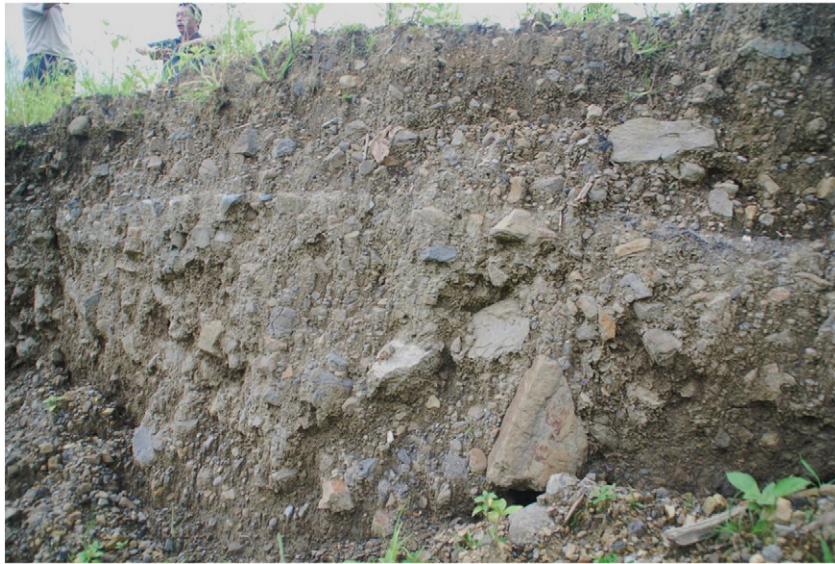
Fig. 1. Cutting slope of typical colluvium in Taiwan.
