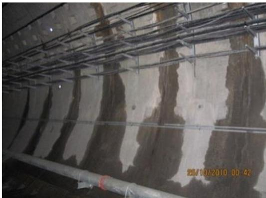
Fig. 1. Leakage of the shield tunnel in low-permeability saturated soils in Shanghai.
