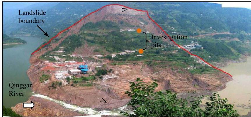
Fig. 2. General view of Qianjiangping landslide (Liao et al., 2005).
