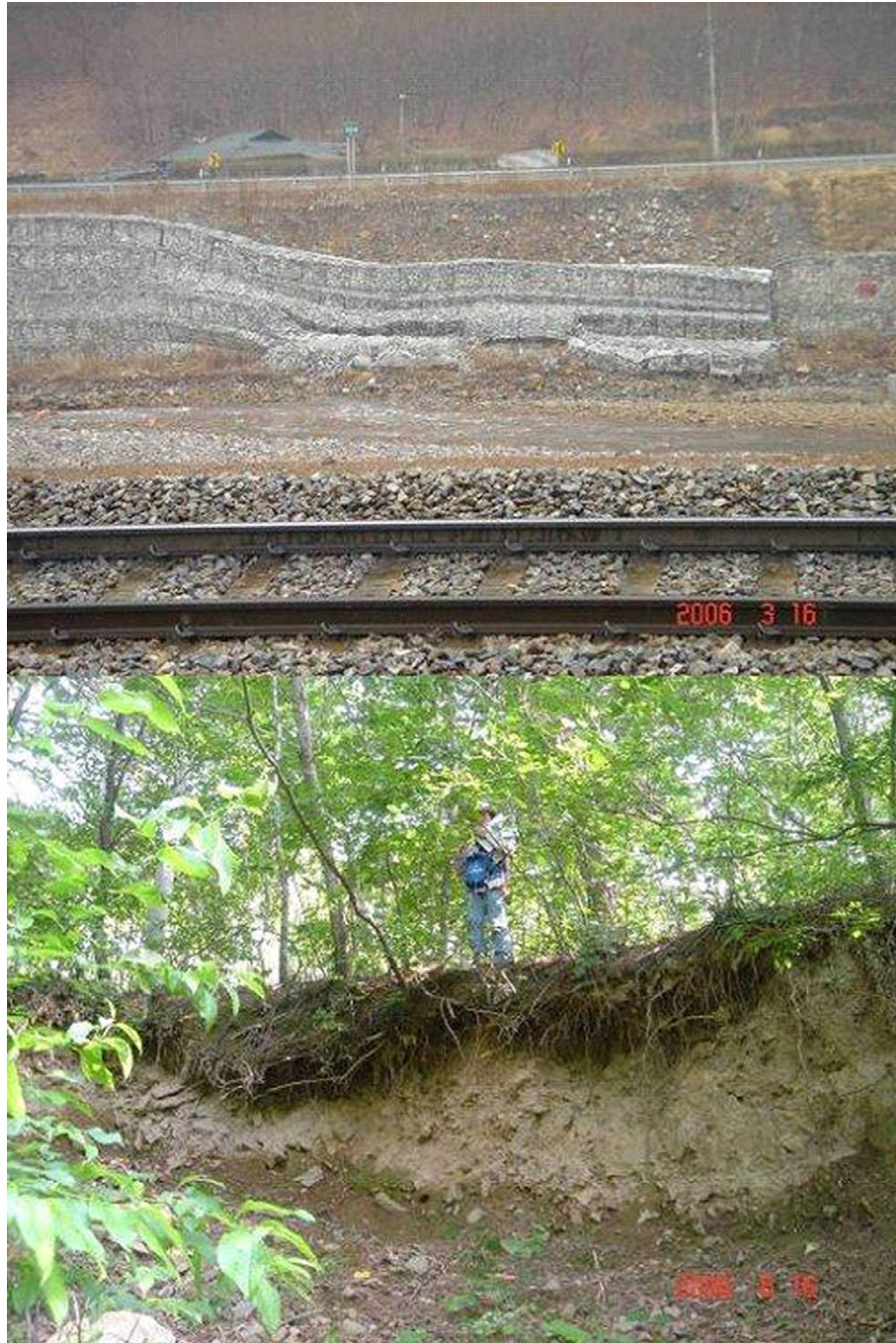
Fig. 1. Photographs of ground subsidences in the study area (above: near railroad, the gabions have bended due to ground subsidence. below: in the field, the ground has sunk by ground subsidence).
