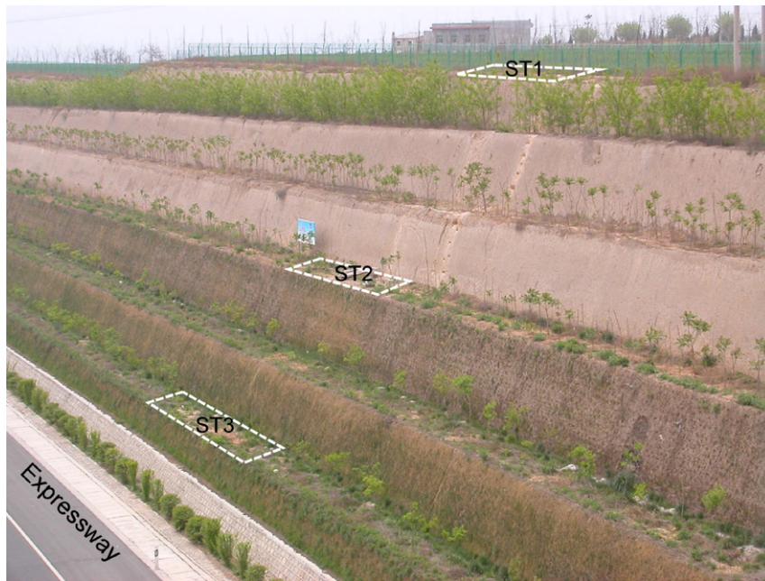
(a) Site photograph showing the monitoring locations on the slope
