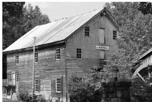
Fig. 2. Cook's Mill, a three-story building, was constructed using hand-hewn logs for the structural framework and covered by clapboard siding. This view is of the northeast corner of the mill and the main entrance is located below the "Old Mill" sign. Laurel Creek, which powered the mill, flows parallel to the south wall.
