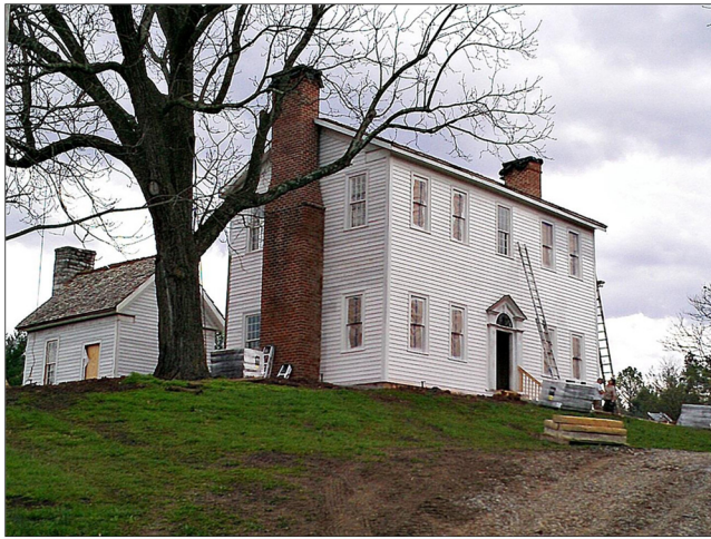
Fig. 1. The historic Sabine Hill house located at Sycamore Shoals State Historic Area in Elizabethton, Tennessee. A weatherboard-covered log pen (left) had been attached to the main house by the “hyphen” room that has since been removed during restoration.
