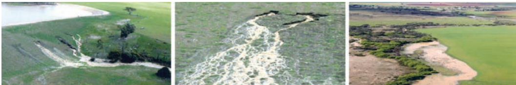
Figure 1: Tunbridge Dam in Tasmania, Australia that experienced failure by internal erosion (piping) and view of evacuated town downstream (Source: Jeffery Farrar (2008) [5])
