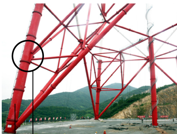
Longitudinal gusset plate connection Concrete-filled CHS member
