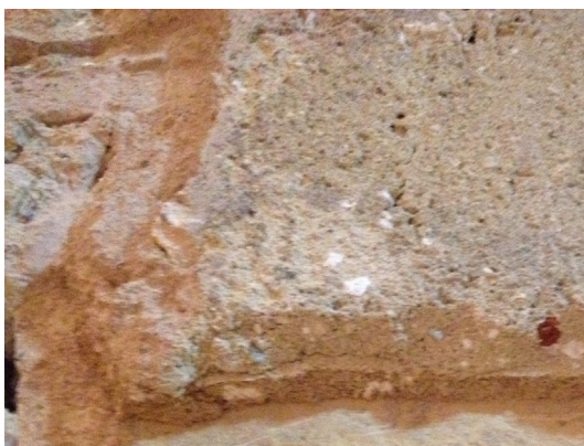
Fig. 2. White lumps in an old air lime render.
