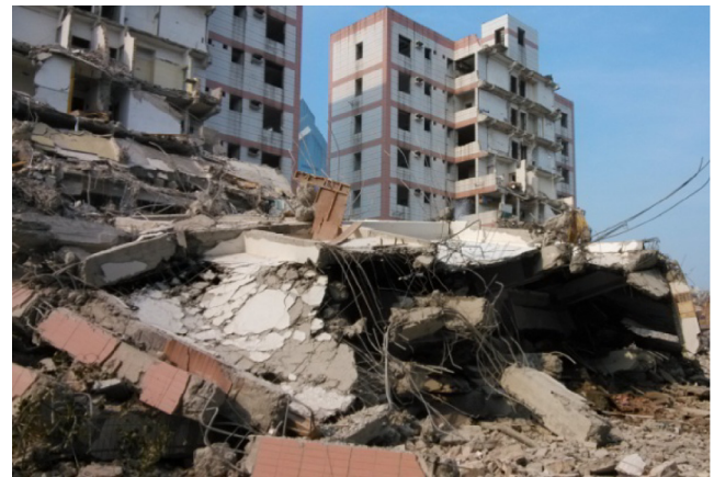
(a) Demolition site
