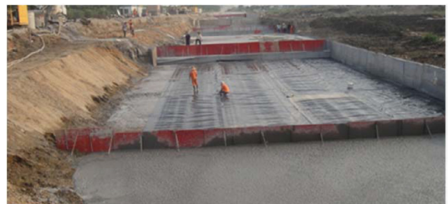
(b) Road subgrade widening
