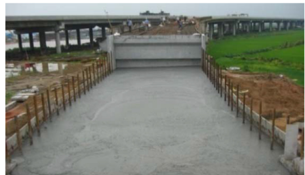
(a) Transition section between bridge abutment and embankment
