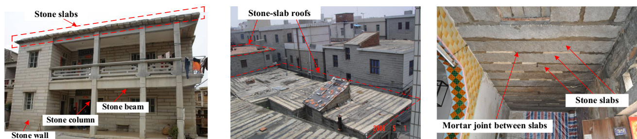
Fig. 1. Stone masonry building in the southeastern area of China.
