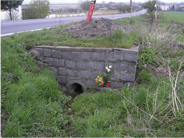
Fig. 1. Example of a cross-drainage culvert.
