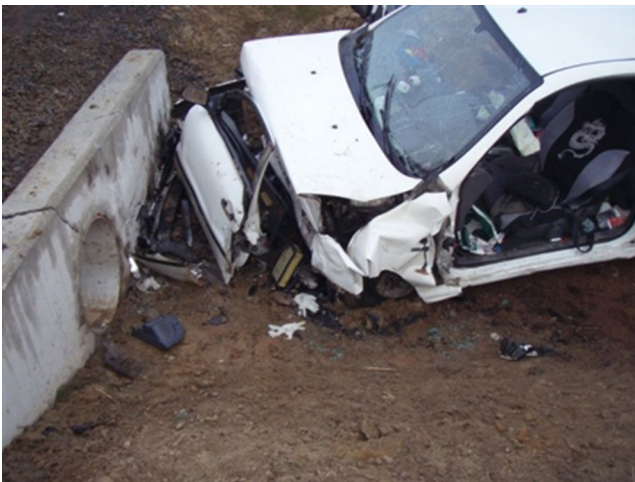
Fig. 2. Collision of a vehicle with cross-drainage culvert.
