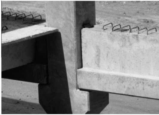
Fig. 1. Application of multi-layers composite inverted T-beam [3].
