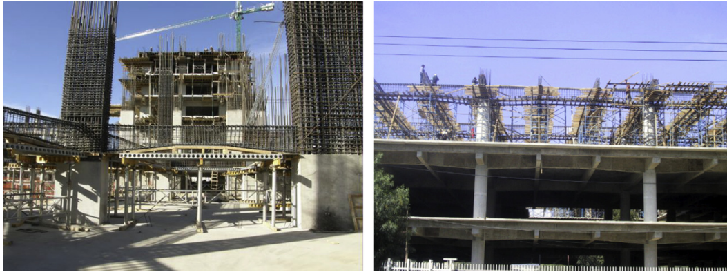
Fig. 1. Examples of buildings with reinforced concrete haunched beams in Mexico City.
