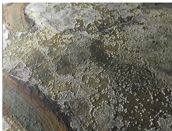
Fig. 5. Polychrome vault: soluble salt crystal aggregates morphology.
