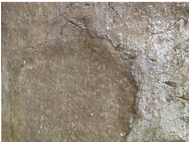
Fig. 3. Sample 1 C. Monochrome wall: white efflorescences are mainly located alongside the border of a patch composed of a different cement mix compared to the surrounding matrix.
