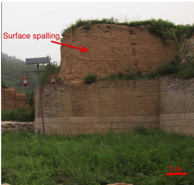
**Fig. 1.** Surface spalling arising from the weathering on the lateral side of the Great Wall.
