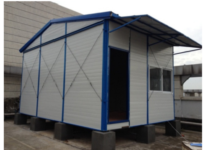
Fig. 2. The photo of the experimental prefabricated house.
