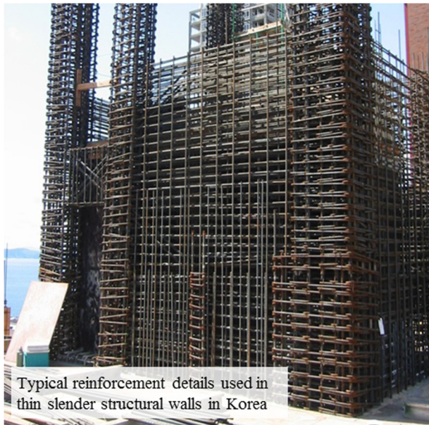
Fig. 1. Reinforcement congestion in thin slender structural walls.
