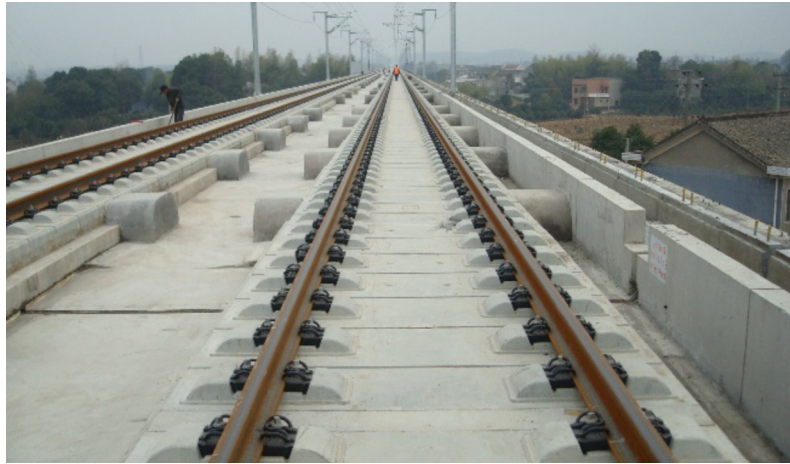
Fig. 1. Ballastless track on a high-speed railway bridge.
