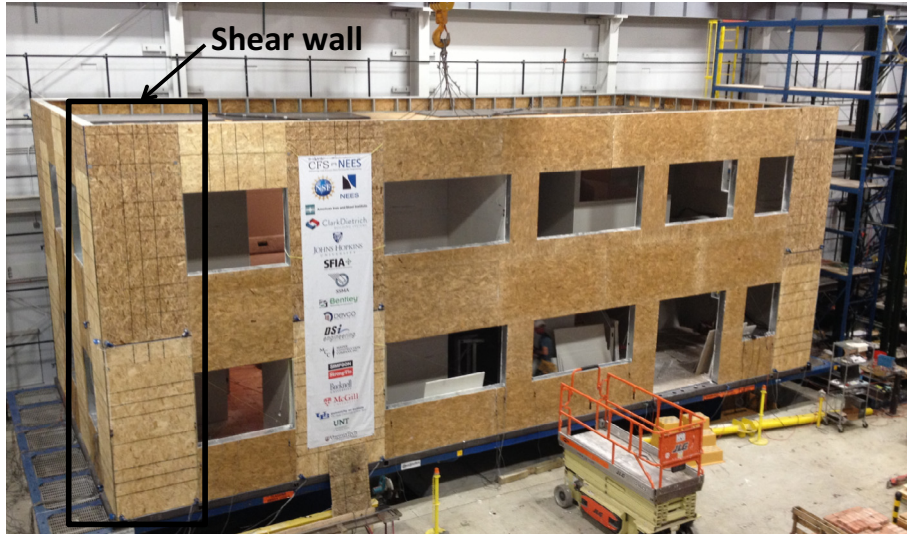
Fig. 1. CFS-NEES building and shear wall in it.
